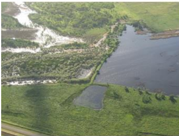
Saltwater intrusion dam constructed across mangrove reaches of lower Kalamia Creek.
