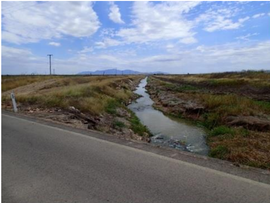
Eroding tailwater drain with dry season riffle flow October 2012 upper Barratta Creek catchment BHWSS.
