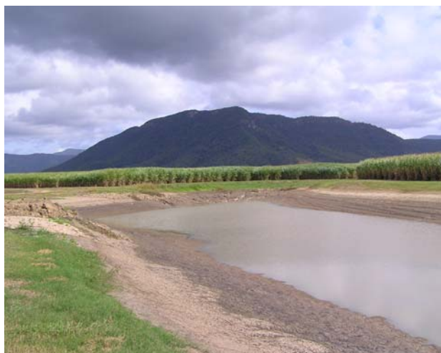
Detention basin acting as both a sediment trap and a sump for a larger ring tank. Photo: QDAFF
