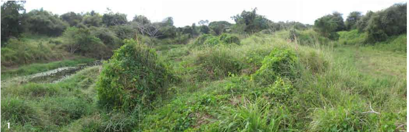
Photo 1: Stuart Lagoon levee bank (photo: Jim Tait)
