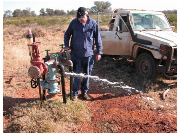
The eastern capped bore. Piping of Wallen's bore water to new watering points facilitated projects to exclude stock from damaged natural waterholes.
