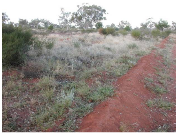
Low banks following contours across erosion prone upland are designed to slow and spread flowing water and promote the return of palatable grasses.
